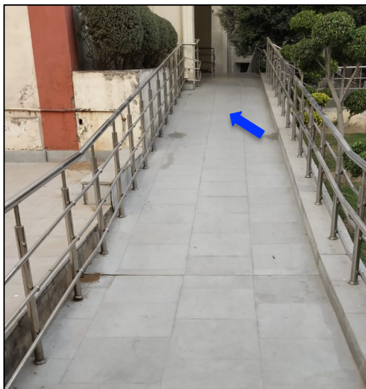
Ramp near the Auditorium
