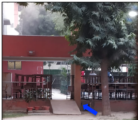
Ramp near the Canteen
