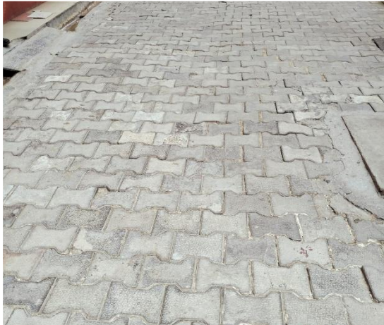
Paving Stone Installed in Campus
